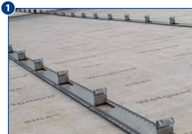
Pre-assembly by means of clip borders or standard clips on a roof surface covered with timber boards and diffusion-open protective sheet
