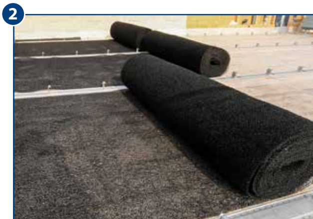
Roll out the structured separating layer as intermediate layer
