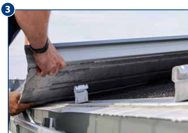
Swivel and lock the RIB-ROOF profiled sheets into the clip border
